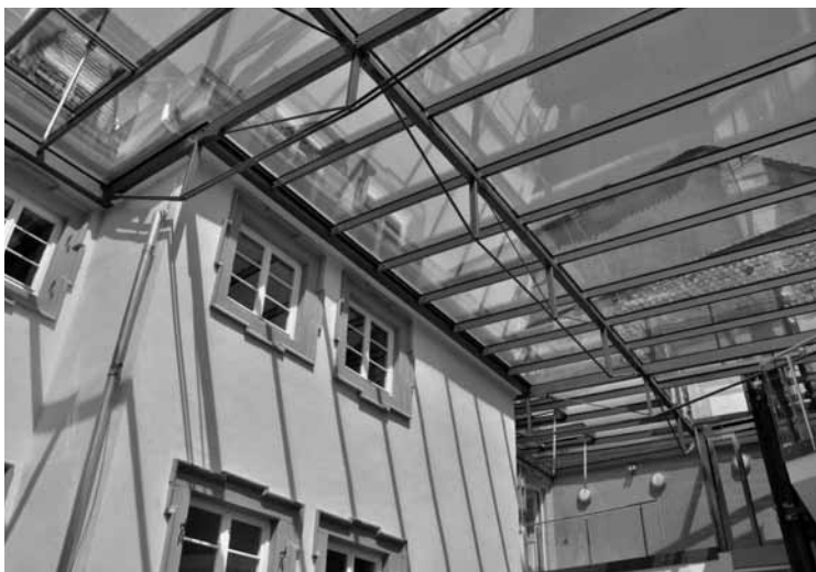
The glass roof of the Atrium.
