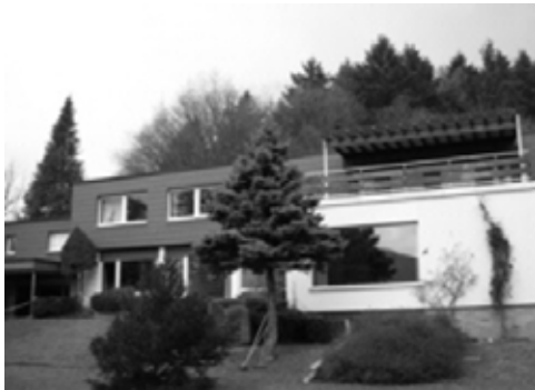
Curt Engelhorn Seminar Center in Oberflockenbach
