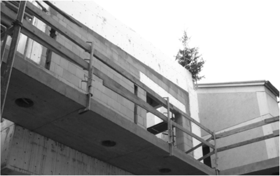
HCA Annex under construction
